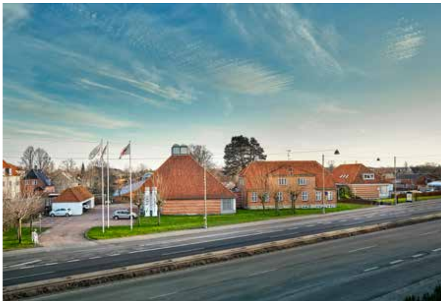
VEKS' Board has adopted renovating and modernising the head office at Roskildevej in Albertslund. Work is expected ready by the end of 2022.
